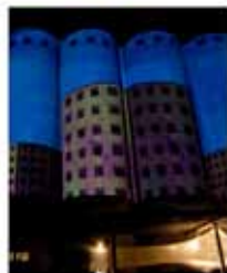
silos - project mikser
